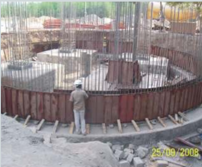
Slip form foundation & Wall form positioning
