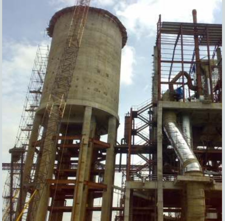
Flyash Silo after completion
