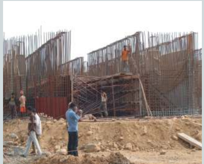
Below deck slab wall for work & bar bending works
