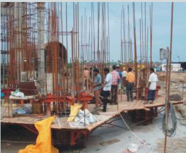
Column slip form assembly at ground level
