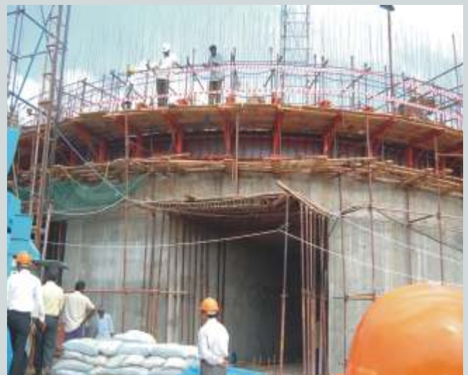
Slip form assembly at deck slab + 5 m level
