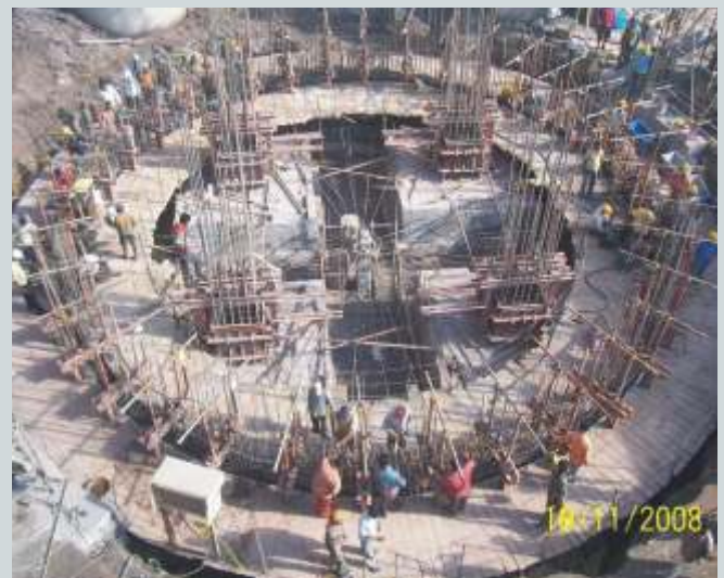
Slip form assembly at (-2m) level both wall & Column
