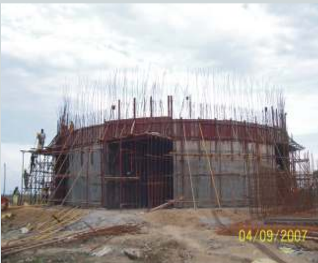
Deck slab concrete works
