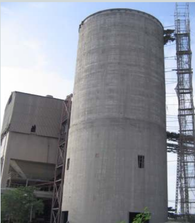
Chilamkur Silo after completion
