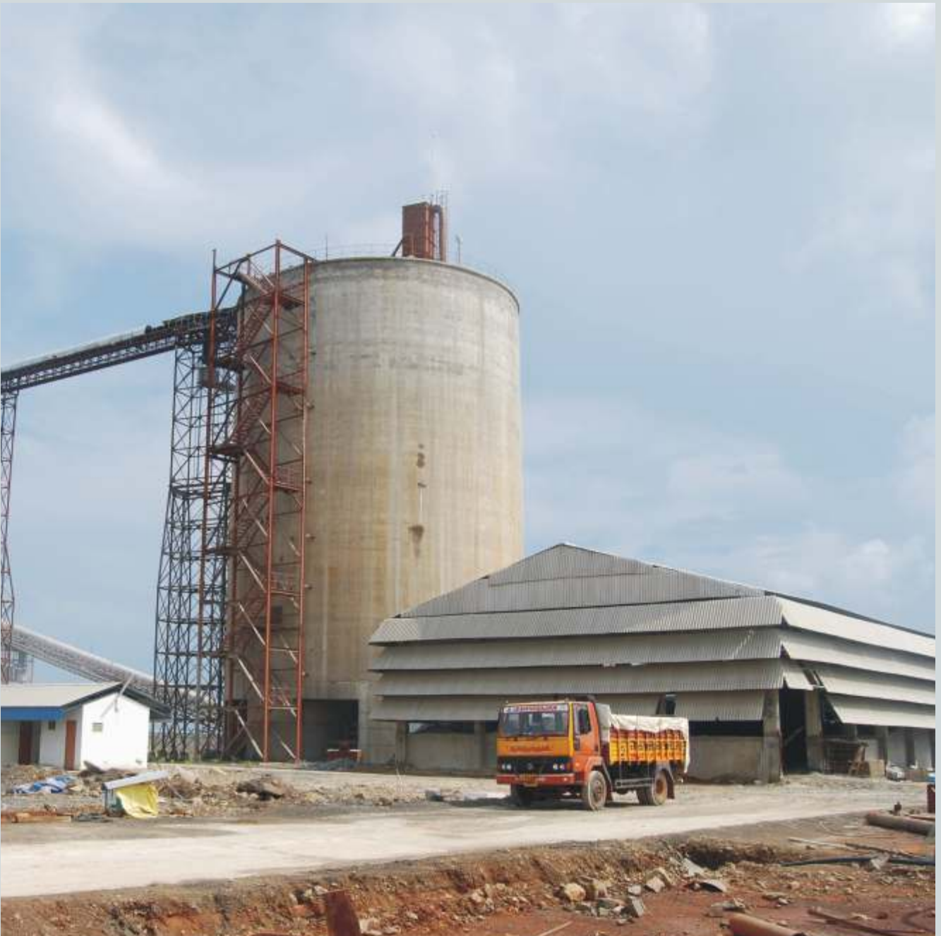
Clinker Silo after completion
