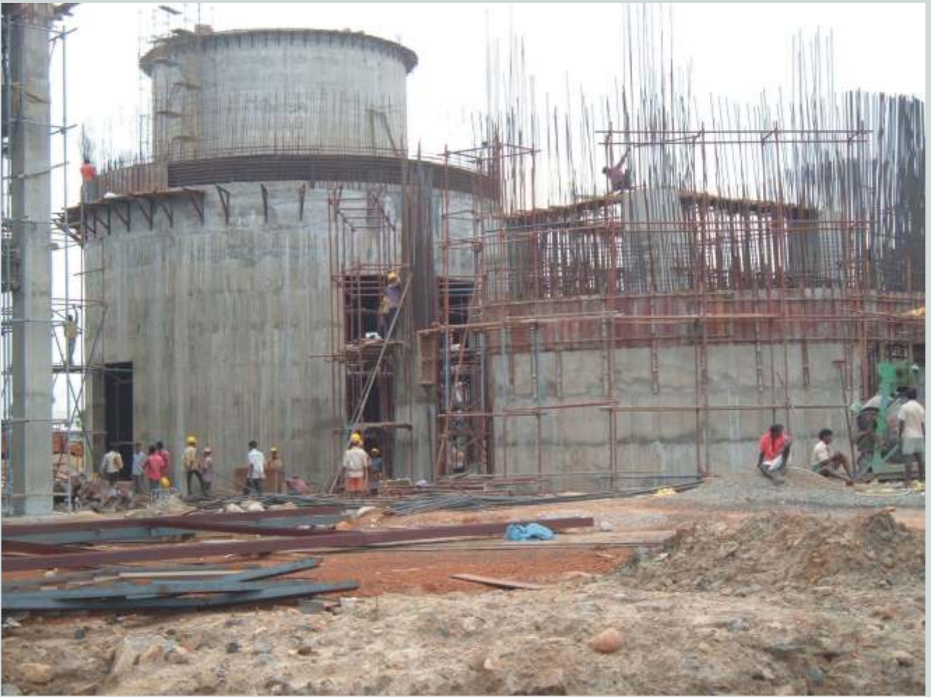
Cement Silo - 2 deck slab preparations
