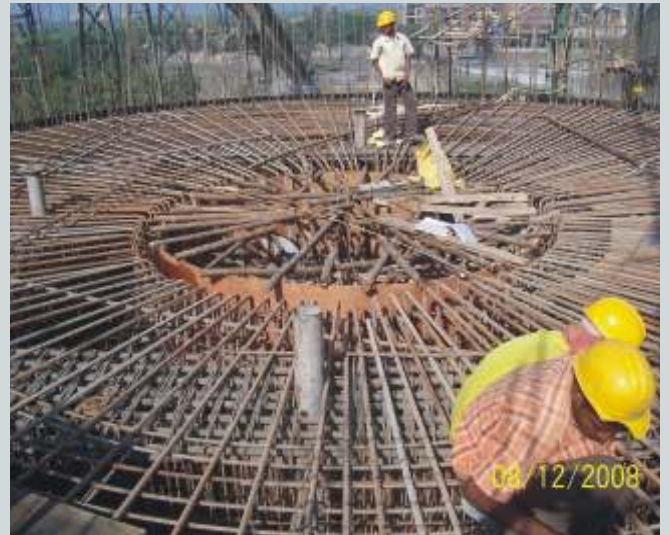
Deck slab form & bar bending works
